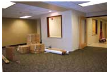
Pictured is the registration and check-out area that will soon be finished and connected to a large patient waiting space for the Trinity Medical Group offices.
