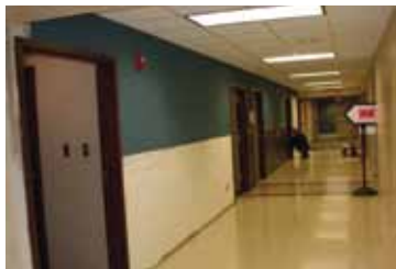
Hallways are brighter as the finishing work is done to the walls and doors in this corridor leading to the Trinity Medical Group Exam Rooms.
