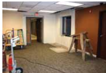
A new registration area and spacious waiting area will soon be opened at the first floor Specialty Clinic. Exam rooms will also be refinished.
